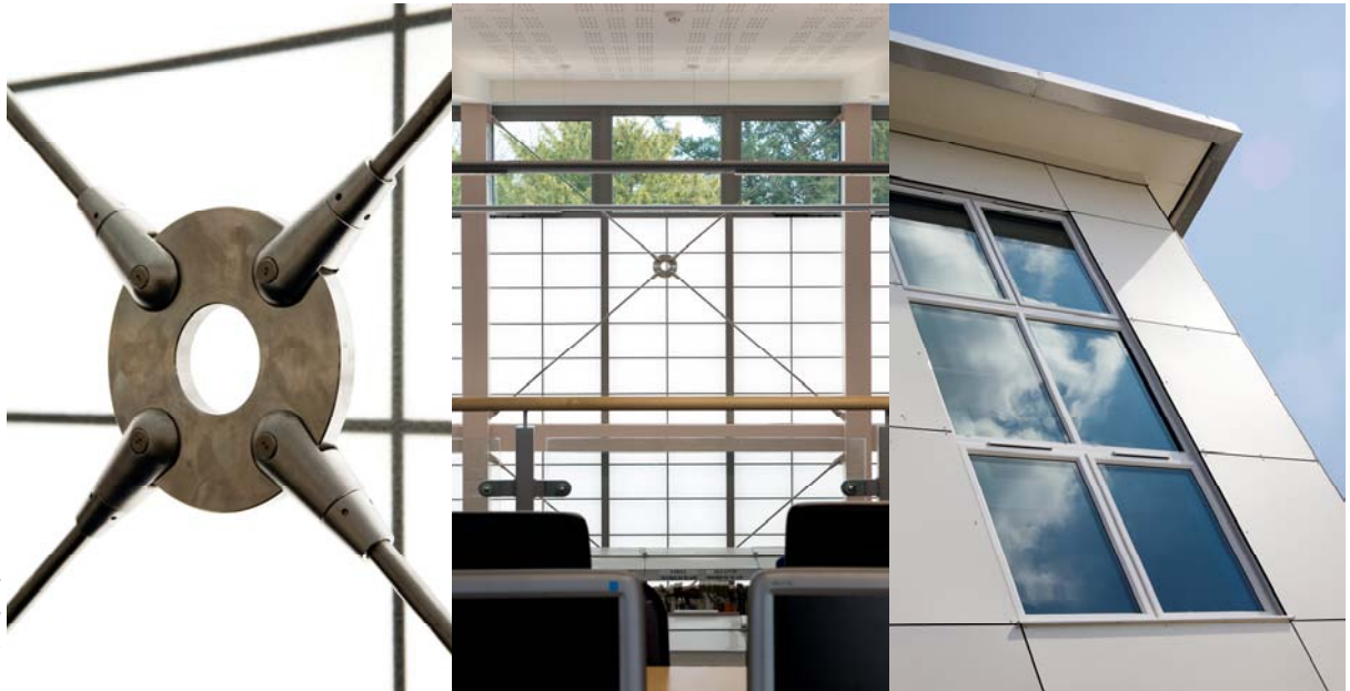
Left to right: images 1 and 2 - the innovative Kalwall translucent bricks, image 3 - part of the new front elevation
